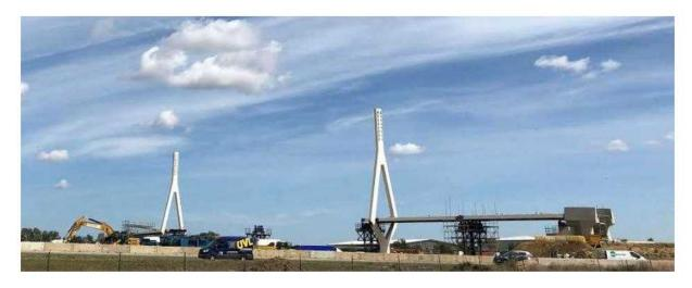
The sections of the deck will rest on the blue temporary supports shown above, while joined to the sections already in place. Eventually the deck will be suspended, as shown in the artist's impression of the finished bridge below.
